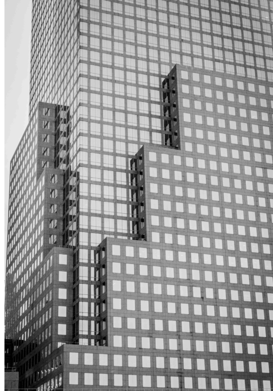
New York, USA. World Financial Center Building.
